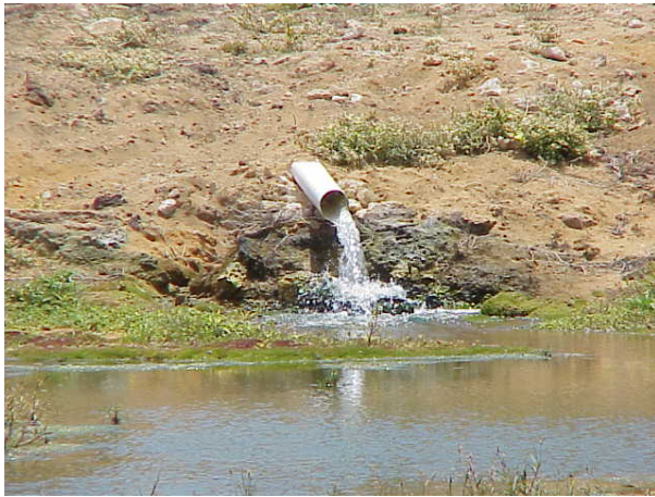
Treated wastewater being discharged to infiltration basins.
