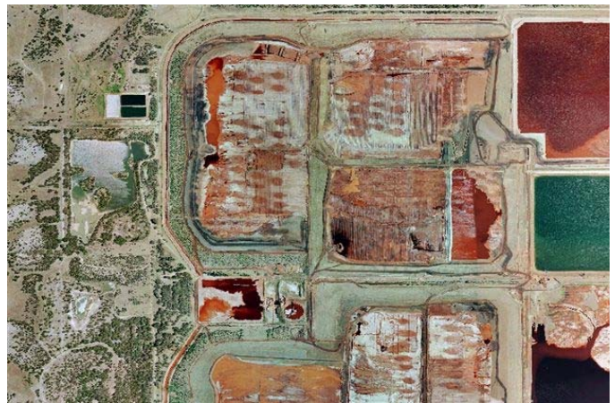
Pinjarra WWTP adjacent to the Alcoa ponds (top left)
