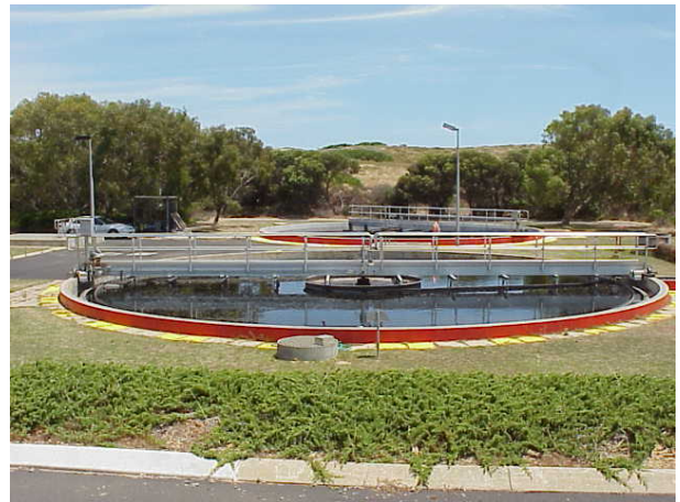
Clarifier settling out solids and producing clear treated Wastewater
